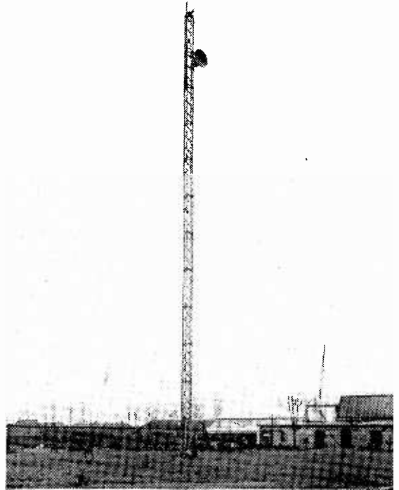
Part of a 200-ft experimental portable mast made of lightweight aluminium alloy to facilitate transport and erection.
